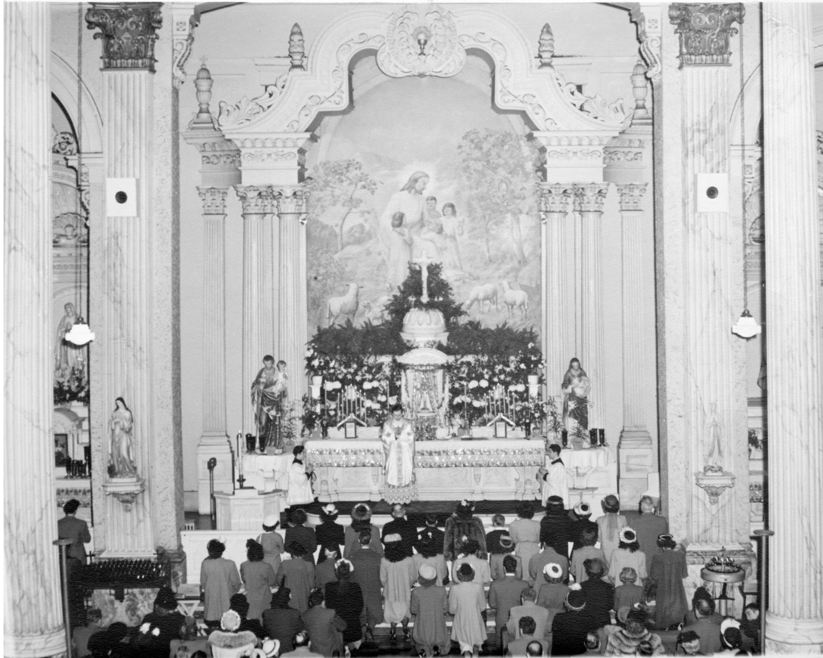
Parish - Photographic Materials - St Patrick sanctuary and altar after renovations circa 1950
