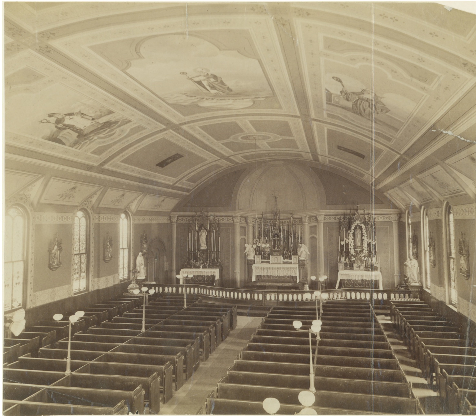
Interior of St. Columbkille's Catholic Church at 8202 Michigan Avenue, Photograph by Emil Boehl, 1890s, Missouri History Museum, N33510
