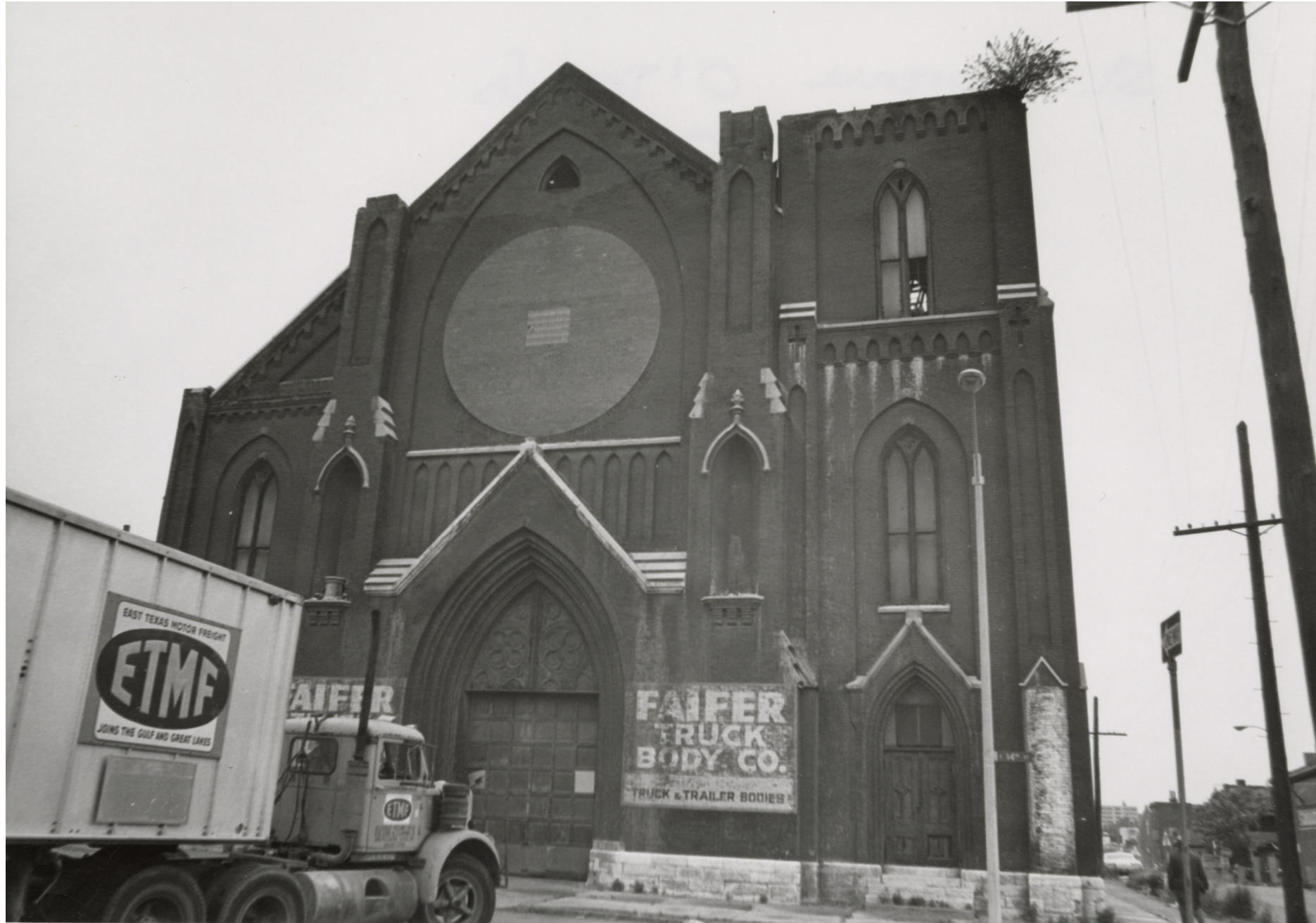
St. Lawrence O'Toole Building, 14 th and O'Fallon, 1971, Missouri History Museum, P0197-S02-00035
