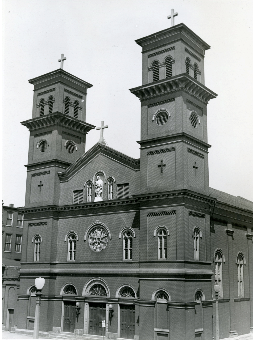
Parish - Photographic Materials - St John Exterior circa 1940
