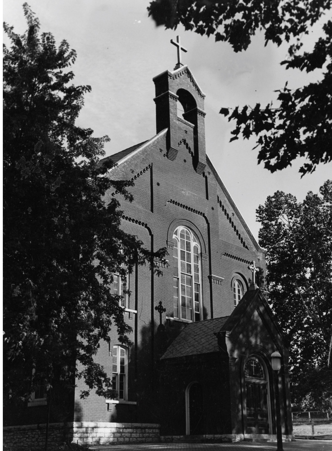
Parish - Photographic Materials - Saint Columbkille Exterior circa 1940
