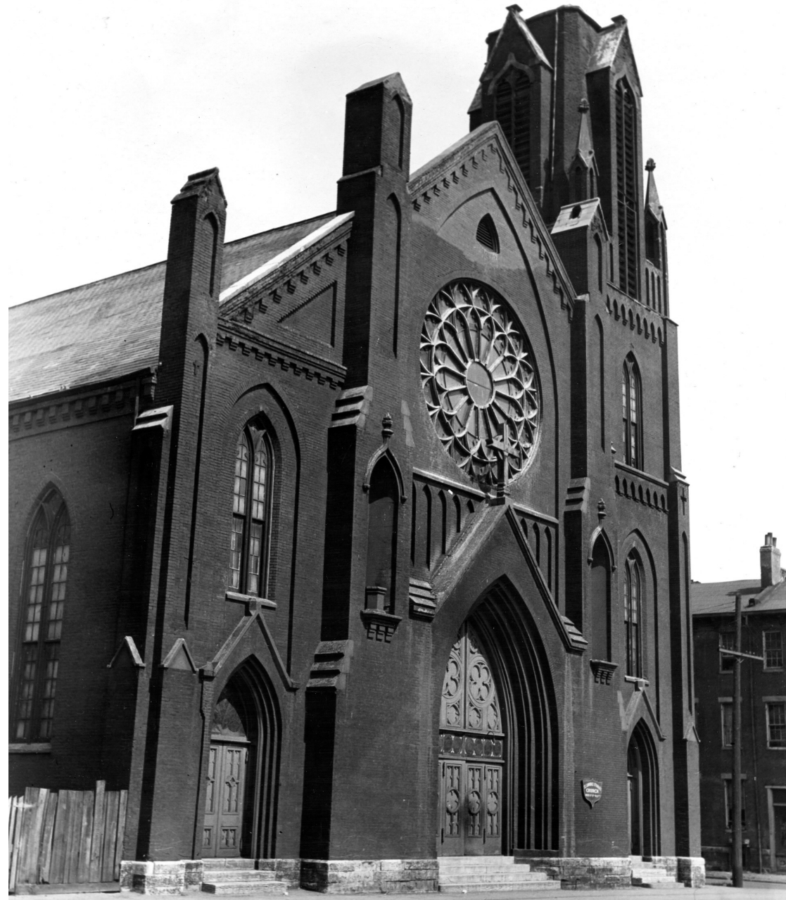
Parish - Photographic Materials - St. Lawrence O Toole Church building, exterior, circa 1940
