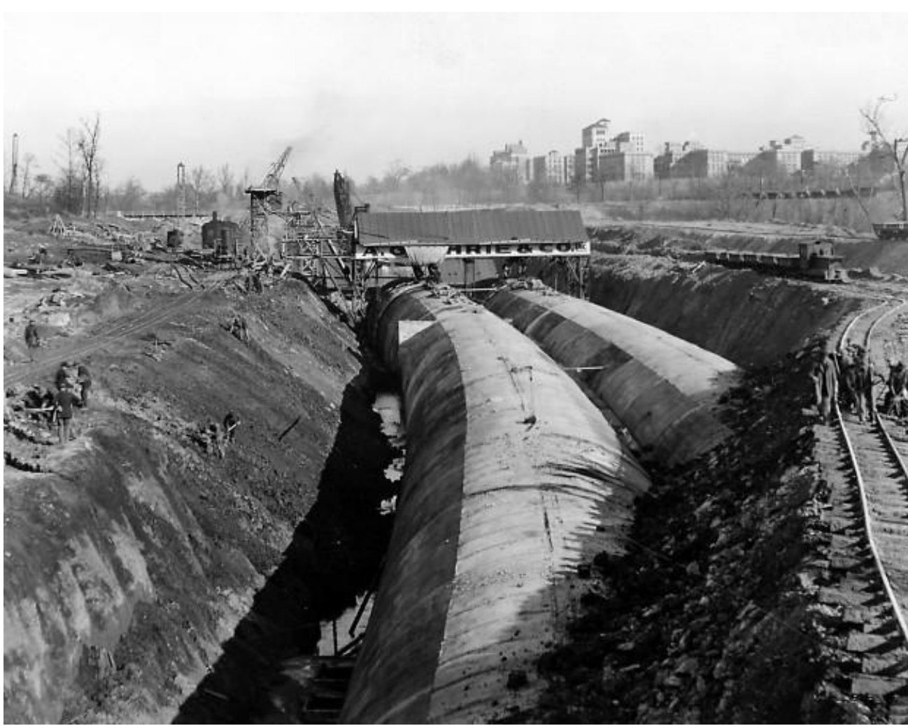
River Des Peres tunnel at Kingshighway
