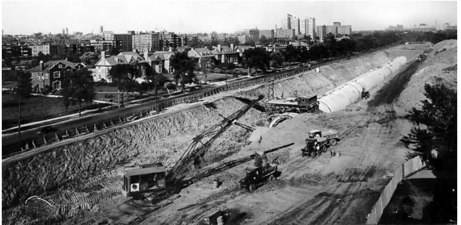
River Des Peres tunnel along Lindell
