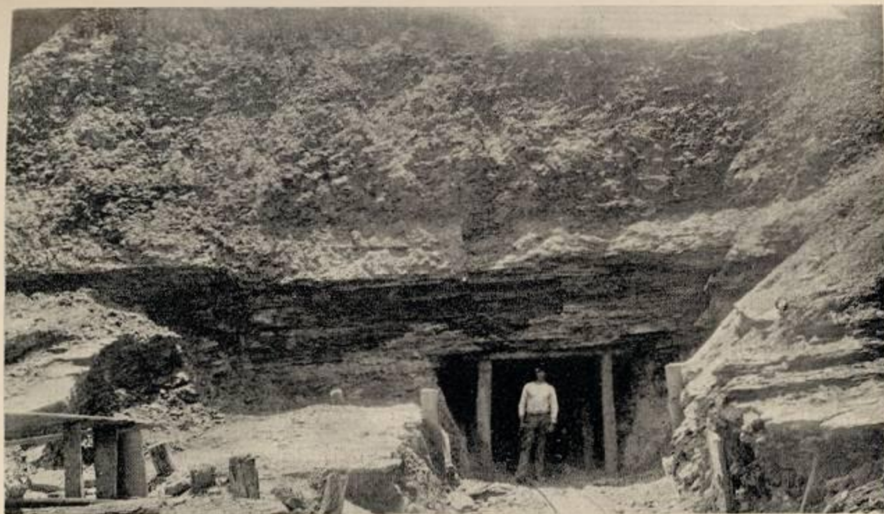
Entrance to the Fire Clay Mine of the Laclede Sewer Pipe Company, showing the sandstone roof and the beds of pipe clay above it.
