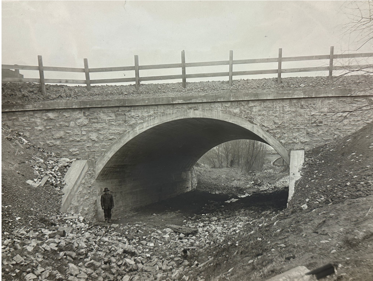
Bridge over River Des Peres at Delmar
