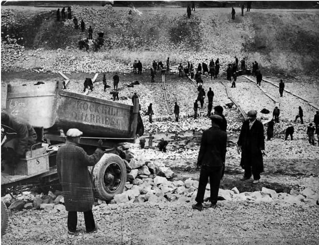
Adding rip rap from Rock Hill Quarries to River Des Peres, 1920s
