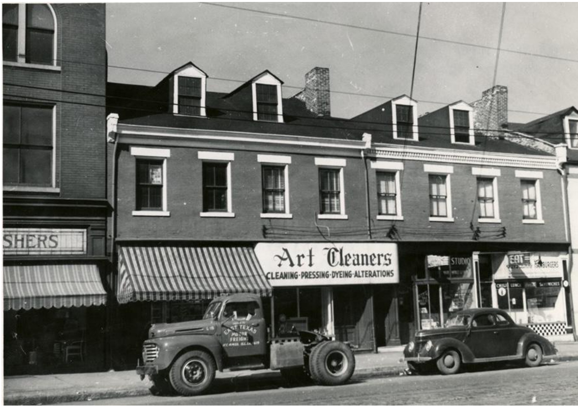
Buildings in front of Wenger Brewery, originally 168 Carondelet Ave, later 1535 S. Broadway.
